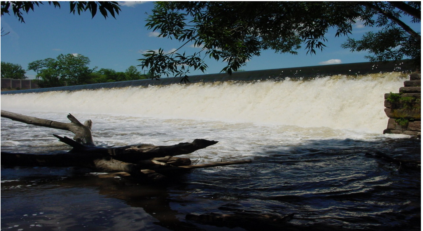
Dundee Dam on the Passaic River
